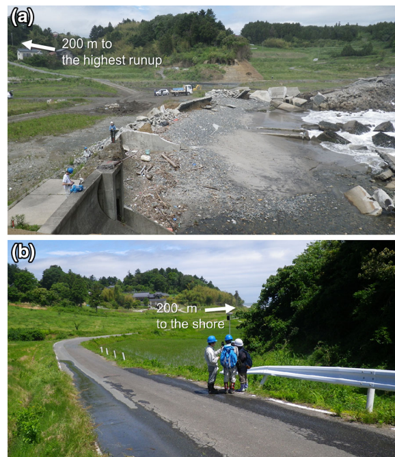
Figure 7 Photos of Kabaniwa, Soma, displaying a completely broken seawall and b location near the maximum runup (June 20, 2012)
