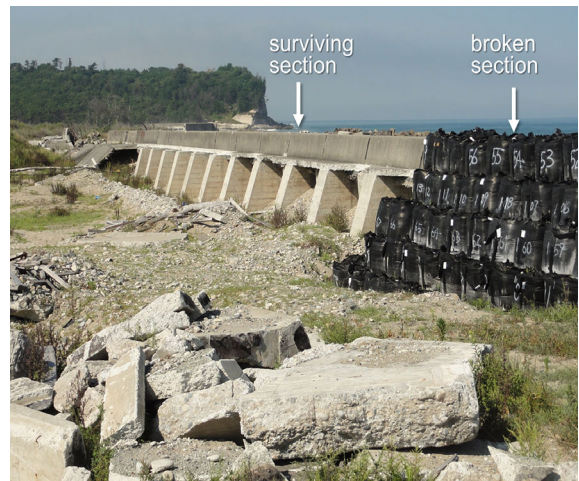
Figure 15 A surviving seawall connected with a completely broken section observed in Naraha (August 24, 2012) approximately 20 km south of the Fukushima Dai-ichi Power Plant
