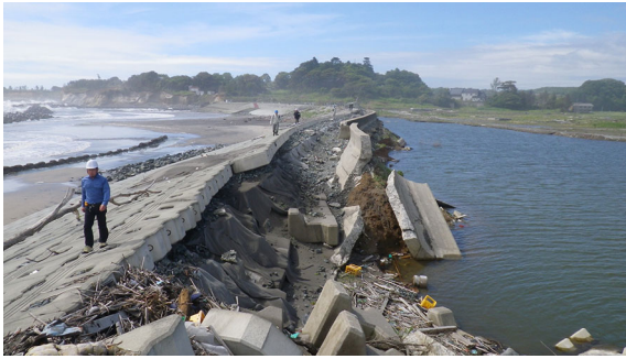
Figure 12 Seawall damage observed in Isobe, Soma (June 20, 2012)
