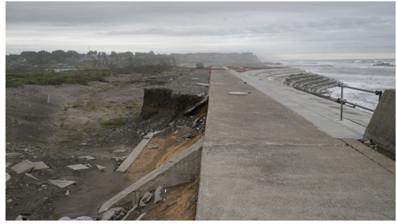
Figure 14 A surviving seawall observed in Tsukabara, Minami-Soma (June 20, 2012)
